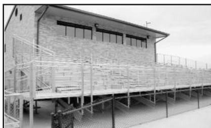
Track & Field Complex
